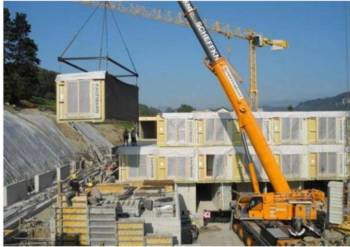
*Figure 5. International best practice in prefabricated timber modules*
