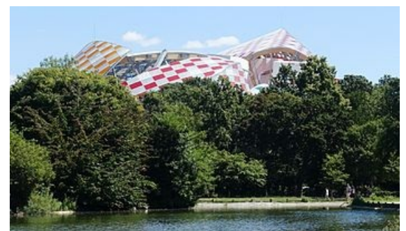
Part of the roof of the Fondation Louis Vuitton building as seen from the Bois de Boulogne in Paris, France (2016)
